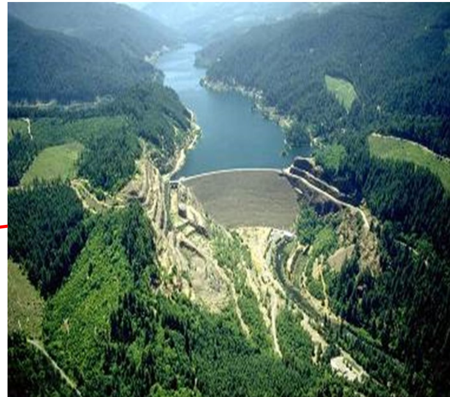
Cougar Dam and Reservoir
